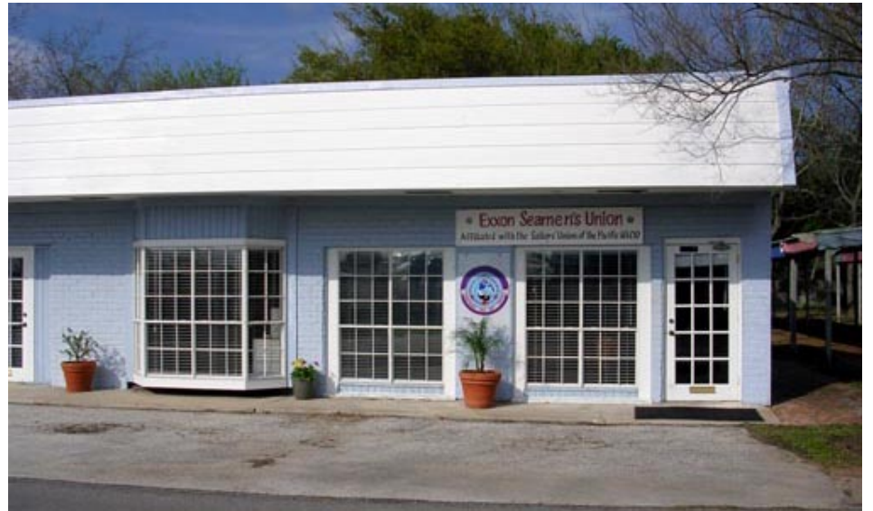
Pictured is the present business office for the Exxon Seamen's Union. The Union settled into its present location at 5 th Street in Seabrook, TX after relocating from Baytown, TX in the fall of 2003. Photo: John Straley
