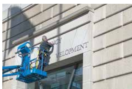
A construction worker removes USAID letters
