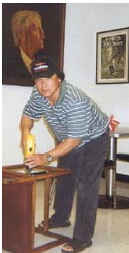
Julian Torre volunteers his time to repair chairs at the Wilmington hall Nov. 11.
